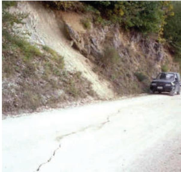
**Fig.2.3.** Fracture cutting the road along the Colfiorito Border Fault at La Pintura.
